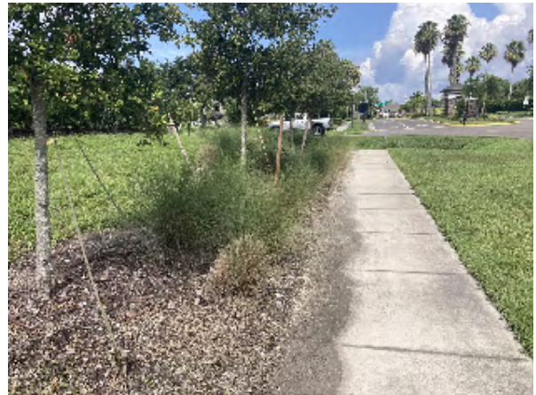
Sidewalk On 11th Street 2
